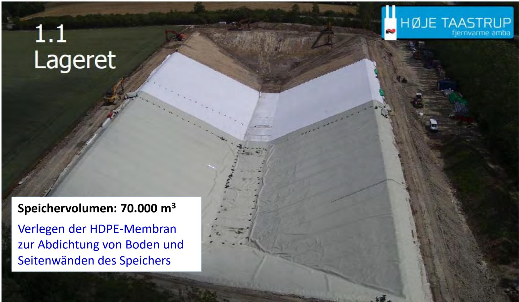
Quelle: Sørensen, P. A. et. al.: FLEX\_TES - Design and Construction of the Pit Thermal Energy Storage in Høje Taastrup. Final Report. PlanEnergi, 2023.
